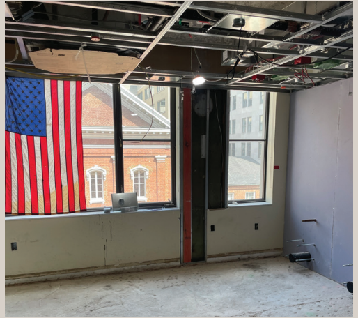
Photos courtesy of Consigli Construction.
